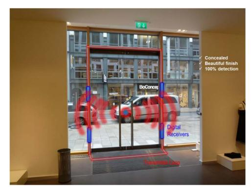
Transmitter can be hidden in the door frame with the controller out of view above the ceiling. The turbo antennas (digital receivers) are mounted in the door frame with low visibility or completely inside the frame.
