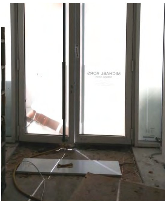
Wi-Fi Floor Guard Antenna prior to pouring concrete
